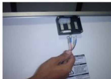
Fig. (i): Opening of module junction box Fig. (ii): Module cable with correct polarity
