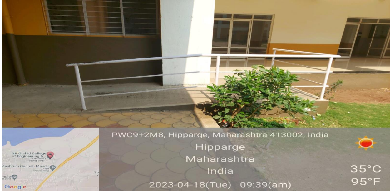
Figure 52: Ramps for Wheelchair with rails
