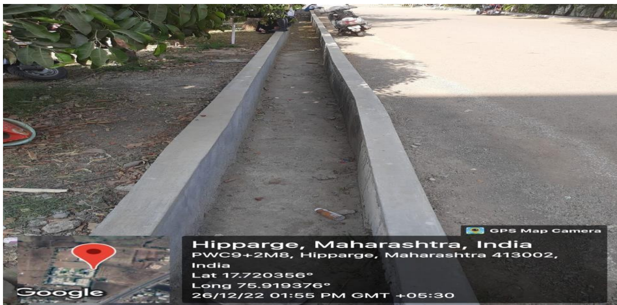
Figure 37: Side drains to collect rain water
