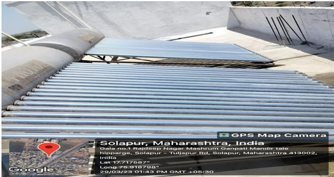
Fig 18: Solar Water Heater installed in Boys Hostel's top floor which helps in reducing electricity consumption
