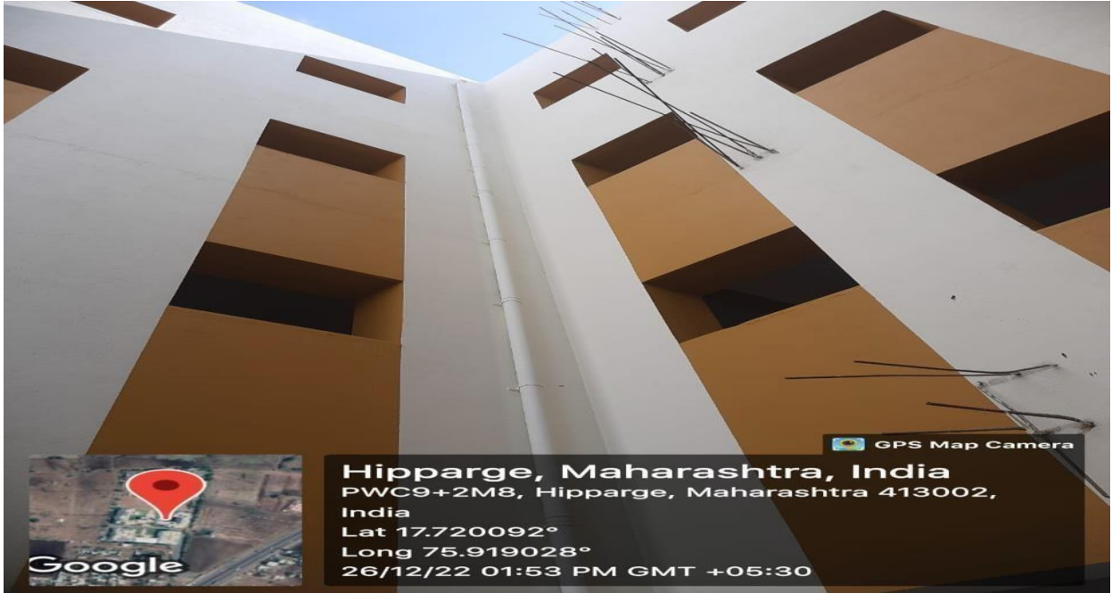
Figure 50: Rain water collected through the pipes is used to water the plants
