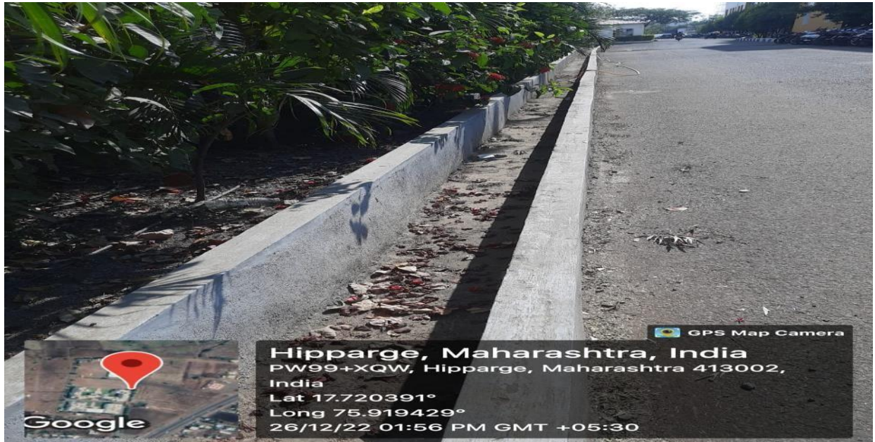
Figure 36: Side drains to collect rain water
