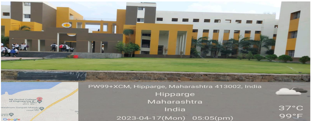
Figure 5: Lawn Sprinkler system operated on Solar Power Generation System
