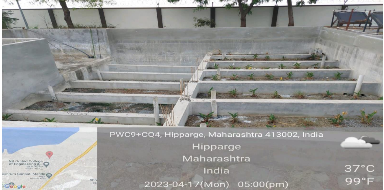
Figure 26: “Recycle and Reuse of Waste Water” (80,000 litre of waste water is treated and reused for gardening)
