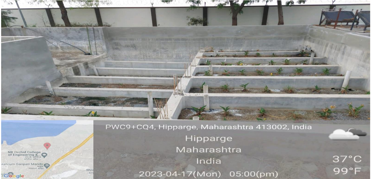
Figure 40: “Recycle and Reuse of Waste Water” (80,000 litre of waste water is treated and reused for gardening)
