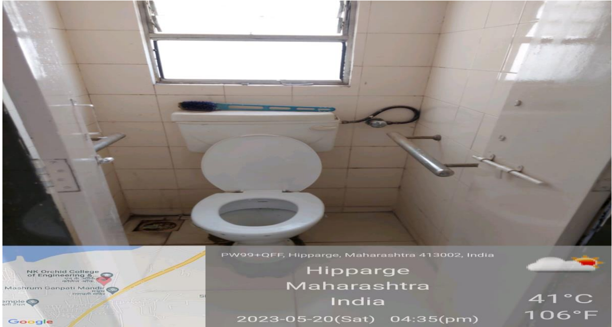
Figure 56: Washroom for the Divyangjan
