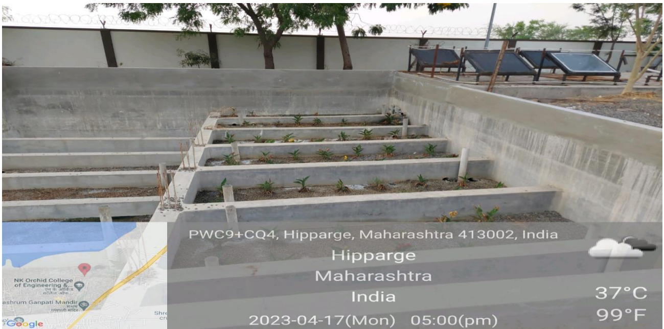
Figure 41: “Recycle and Reuse of Waste Water” (80,000 litre of waste water is treated and reused for gardening)
