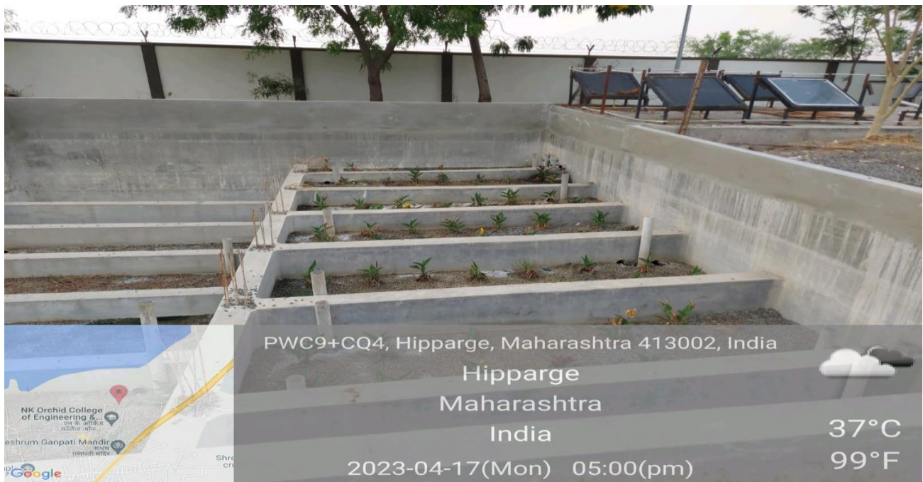
Figure 27: “Recycle and Reuse of Waste Water” (80,000 litre of waste water is treated and reused for gardening)
